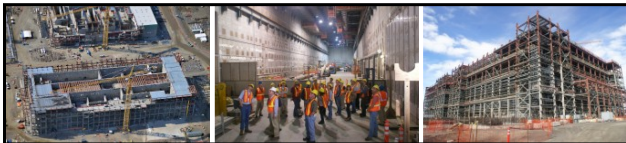
Fig. 1. Pretreatment Facility Construction.
